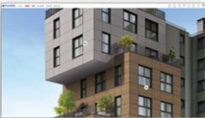
Multi-storey residential building
