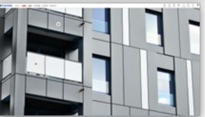
Balconies and parapets
