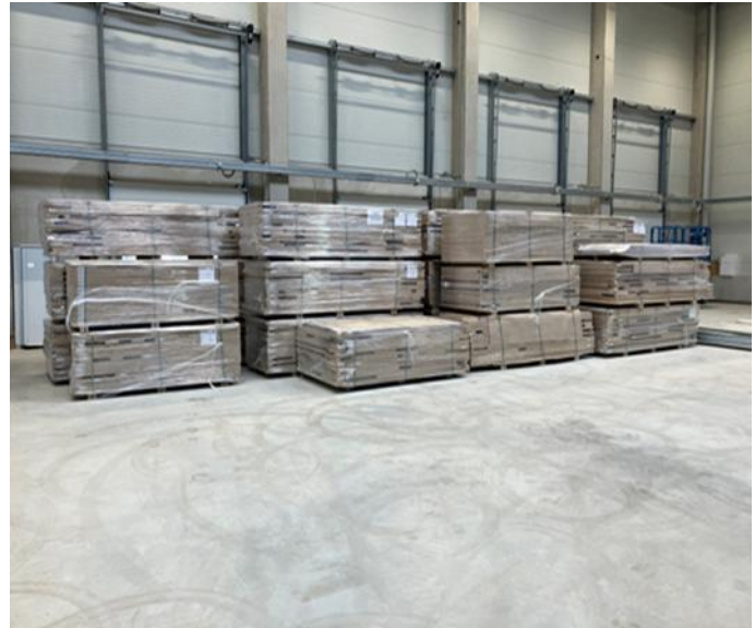
Image 3: Correct storage on site
